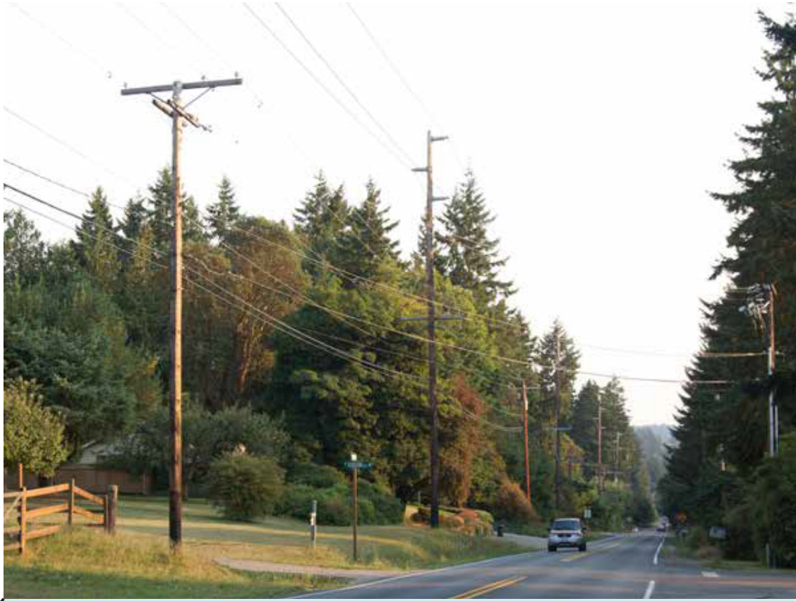
Transmission lines above distribution lines on Madison Avenue NE
