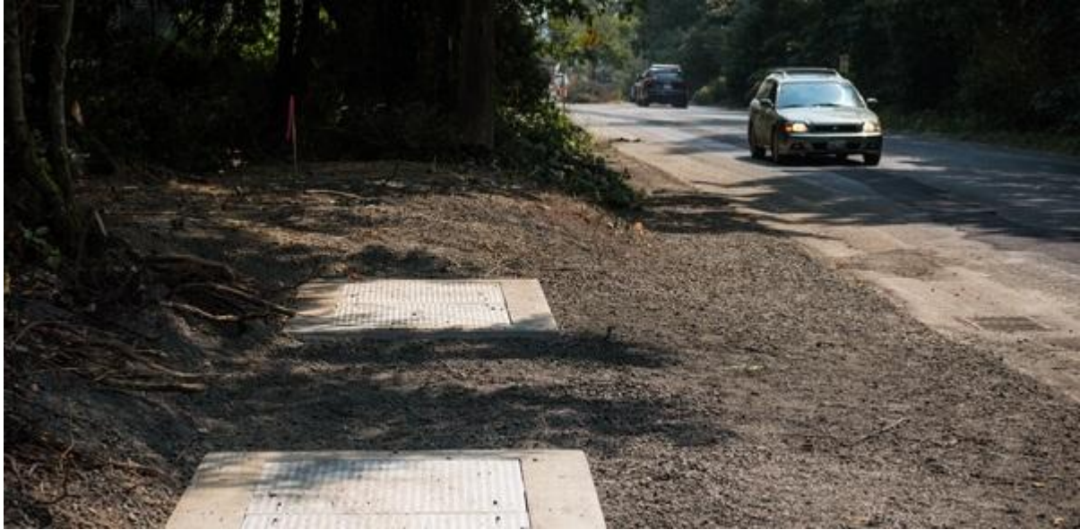
Completed underground vaults along Blakely Ave NE.
