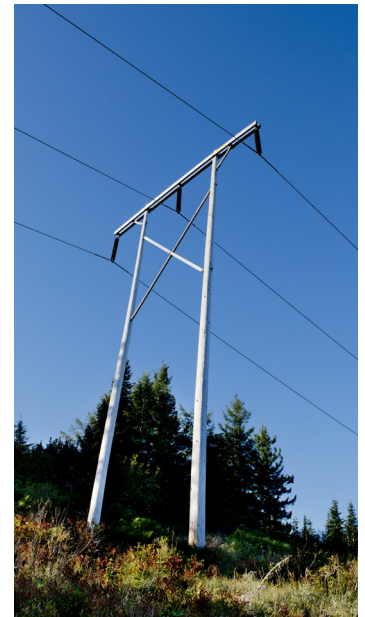
230kV transmission lines
